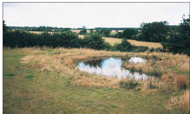
The completed pond in the following summer
