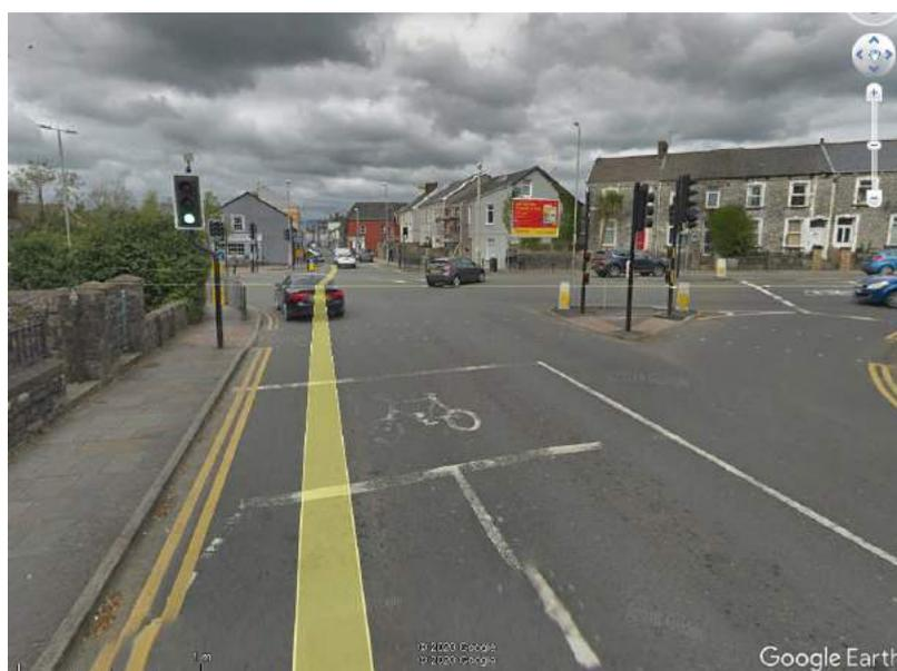
Image 15 – Advanced cycle stop line at Ewenny Rod/A473 traffic signals (all arms). Lining fading. Pedestrian crossing phases incorporated in the signals (north, west and south arms). (© Google Streetview 05/18)
