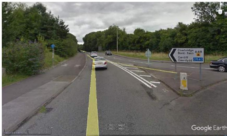
*Image 1 – Shared Cycle Path, dropped kerbs and tactile paving crossings at Broadlands Roundabout facing east along A48 (© Google Streetview 08/16)*
