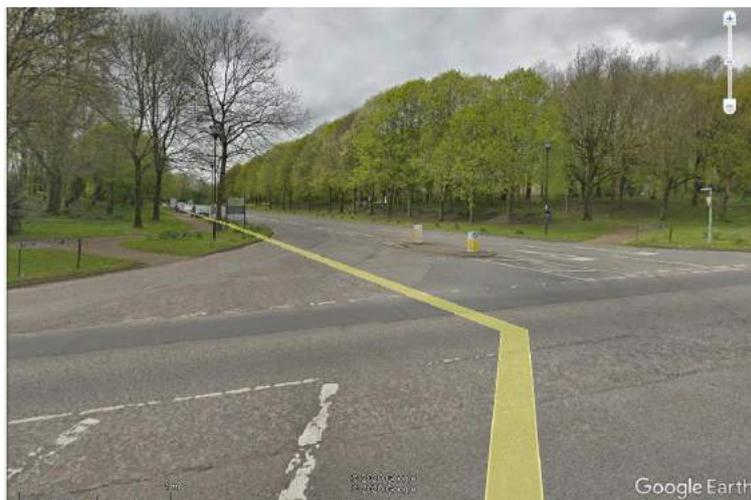
*Image 18 –Dropped kerbs and pedestrian refuge island at Technology Drive. Tactile paving absent. (© Google Streetview 05/18)*
