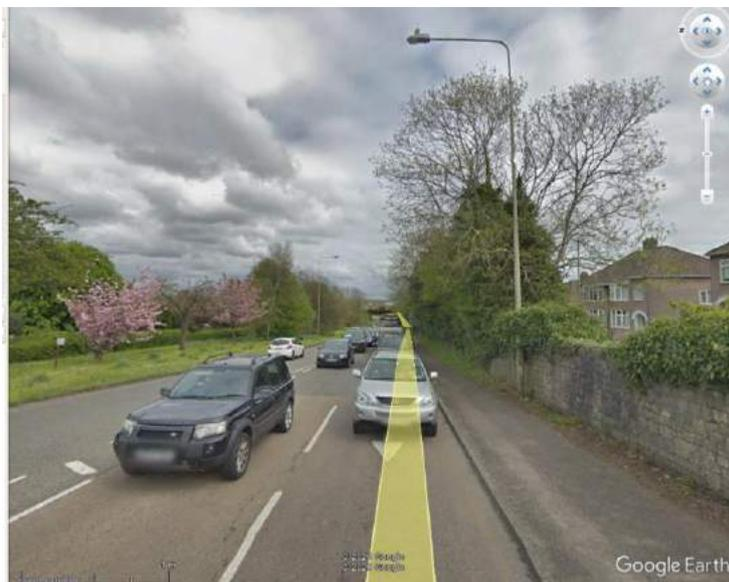
*Image 22 – Street lighting present. Footway narrows on southern side of A48. There is potential scope for widening to create a shared pedestrian/cycle route (© Google Streetview 05/18)*
