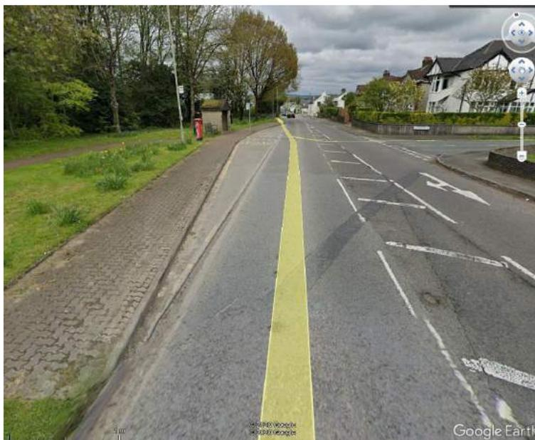
*Image 20 – Tactile paving absent from Priory Avenue junction. Footway of an acceptable width commences on western side of Ewenny Road (© Google Streetview 05/18)*
