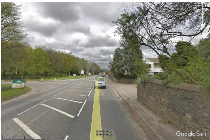
*Image 19 – Tactile paving and dropped kerbs absent from eastern access. Footway on eastern side is sub-standard (too narrow) (© Google Streetview 05/18)*
